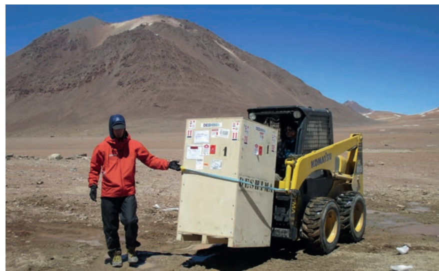
Figure 3. Transportation of the DESHIMA cryostat for installation requires a lot of care to avoid mechanical shocks.
